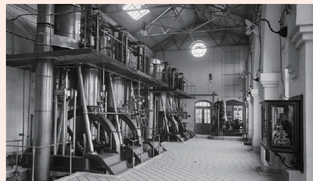
Steam pump at The Onga River Pumping Station during operations
