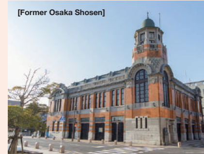
[Former Osaka Shosen] The Osaka Shosen Moji Branch, built in 1917 (Taisho six), has been restored. The first floor now houses the "Watase Seizo Gallery."
