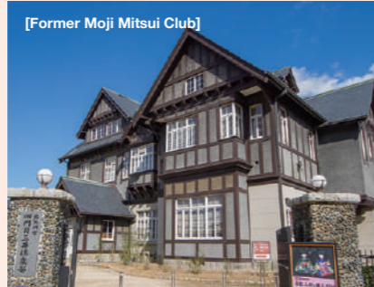
[Former Moji Mitsui Club] Built in 1921 (Taisho ten) as Mitsui & Co.'s social club, this building was constructed using traditional European wooden construction methods.
